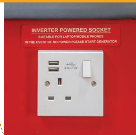
Inverter powered socket c/w USB is located in seating area
